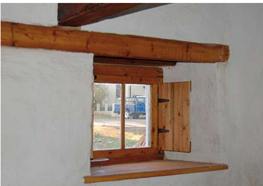
This casement with wooden sill shows how thick the old clay walls were
