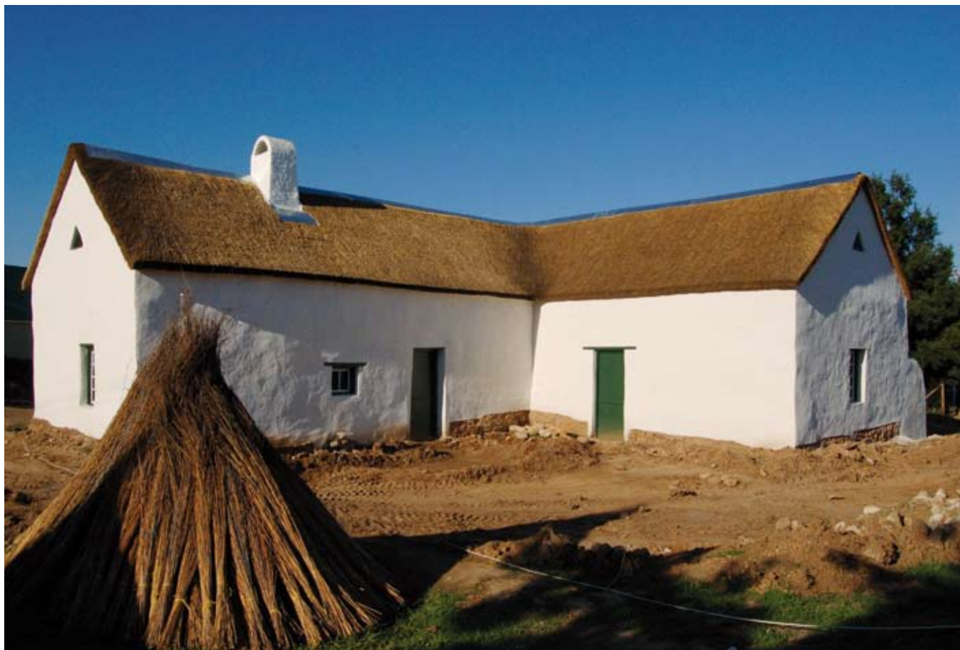
Fourie House in June 2007, with its new thatched roof and lime-washed walls. The front of the house faces away to the right; the left-hand part is the leg of the T, comprising the original kitchen and storeroom
